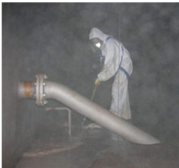
Tank cleaning prior to internal inspection
