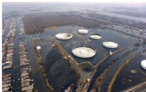
Murphy oil spill, New Orleans, Hurricane Katrina (2005)
