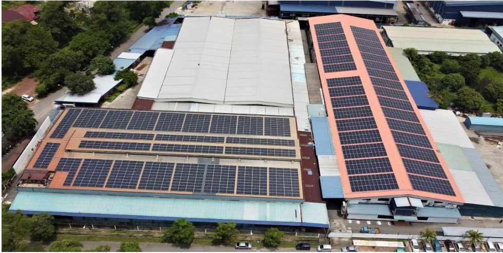
Electronic Manufacturing – Penang (2.8MWp)
