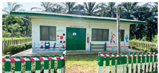
Workers housing and childcare centre at a Sabah estate.
