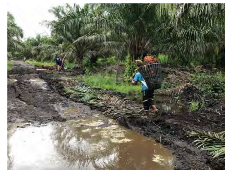
Badly rutted road in Sg Mangga Estate.
