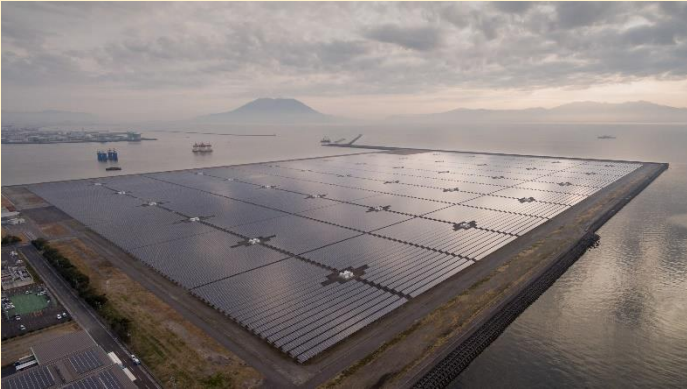
The 70 MW Kagoshima Nanatsujima solar power plant on the south coast of Japan was built in 2013 following the Fukushima nuclear disaster. It is an example of the FiT scheme benefitting Japanese solar. (Image © Christian Åslund / Greenpeace)
