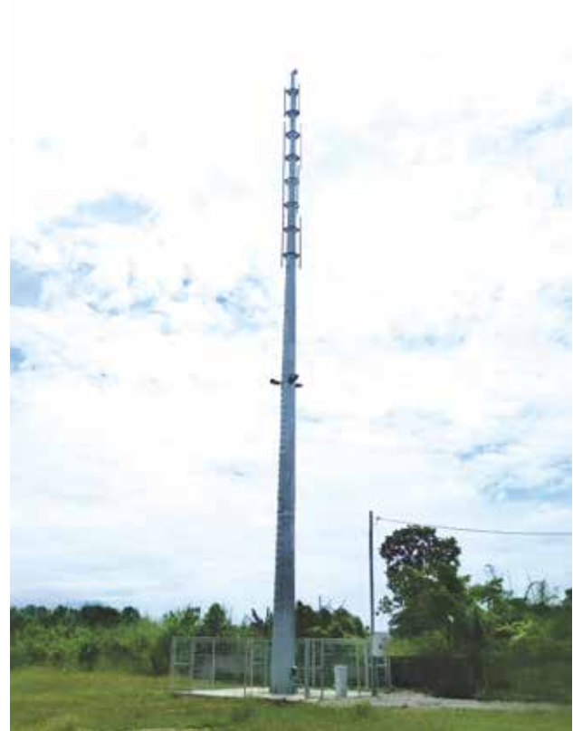
The 30m Telecommunication Tower erected in Kg Paya Berenjut, Kemaman, Terengganu.
