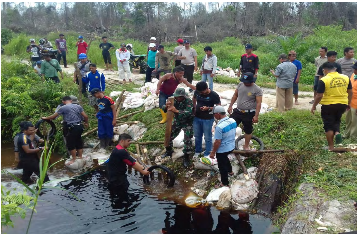
Employees undertaking canal blocking exercise together with the local police at one of our estates in Riau, Indonesia
