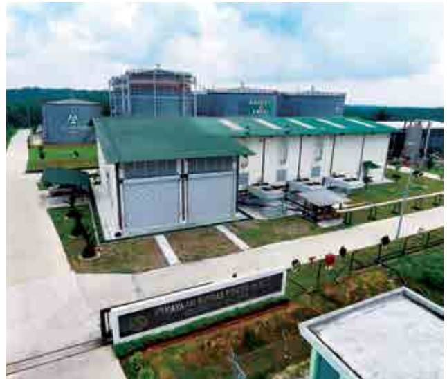
Kekayaan Biogas Power Plant in Johor, Malaysia.
