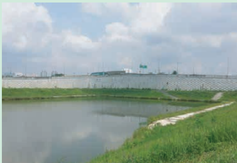
Kolam takungan banjir Puah, Selangor
