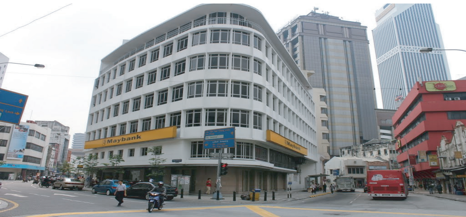
Maybank, Jalan Tun H.S Lee
