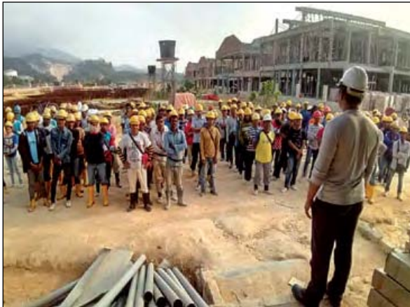
Tool Box Meeting At Our Project Worksite
