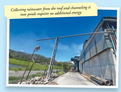
New gutters are installed to collect and channel rainwater to the collection ponds.
