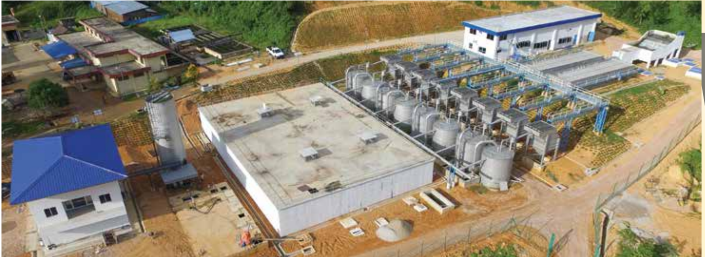
23 MLD Surface Water Treatment Plants in Pahang, Malaysia.
