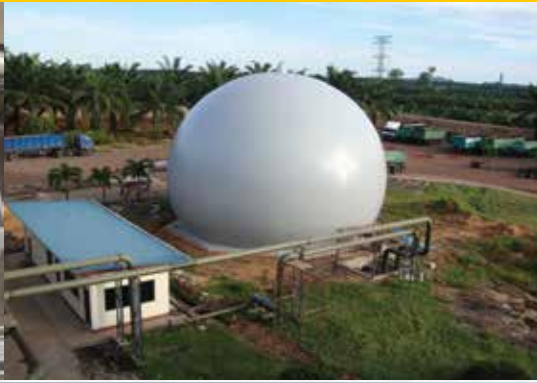
Double Membrane Gas Holder, Sabah
