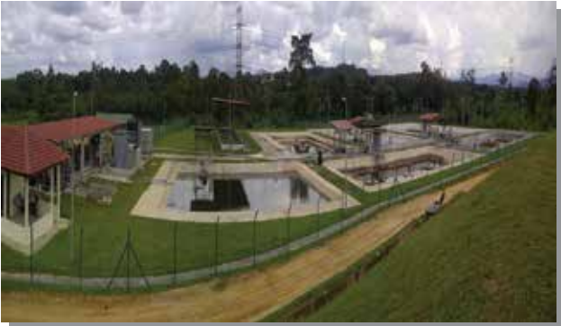
Leachate Treatment Plant
