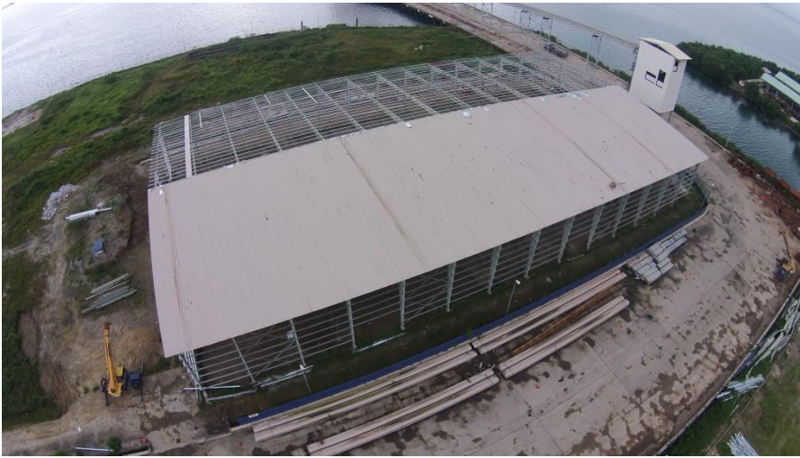
General cargo – PKE/PKS warehouse
