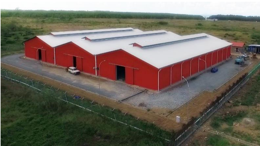
Biomass Collection Warehouse
