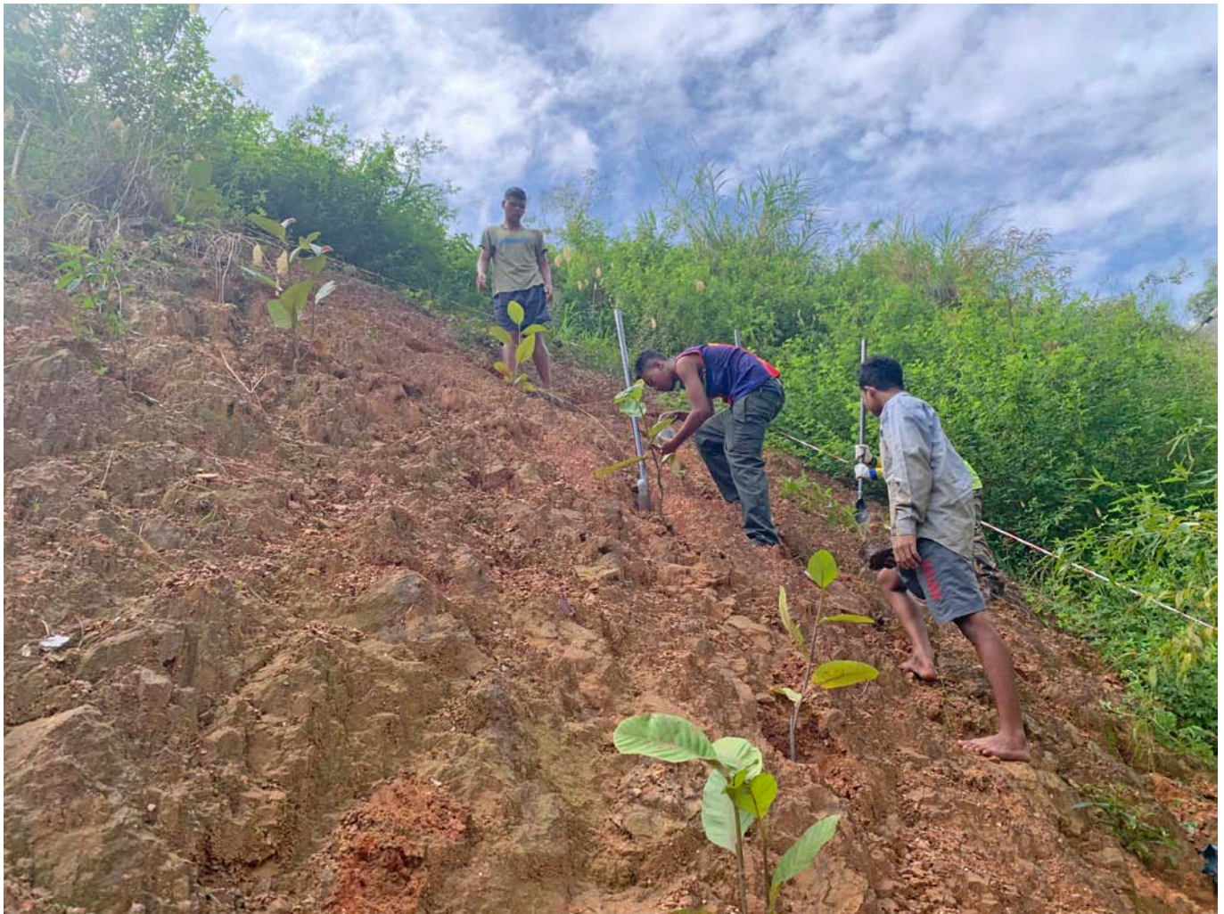
Trees that heal: The planting of suitable tree and plant species helps establish a natural and stable ecosystem to prevent soil erosion next to the Simpang Pulai - Cameron Highlands highway; with most tree species planted achieving 100% survival rate.
