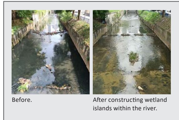
The introduction of wetlands islands helped improve biodiversity and enhance selected water quality parameters of targeted stretch of river. The initiative also saw a school of fish coming back to this particular stretch.
