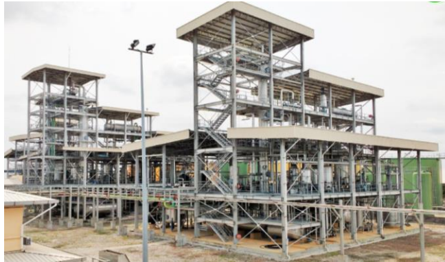
TPG Oil & Gas (80.0% subsidiary of CBIP)
