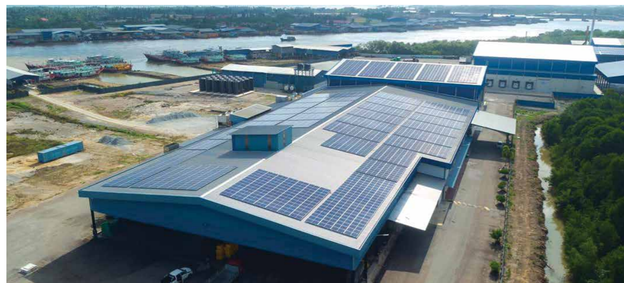
Solar panels installed on the roof of our plant at Endau, Johor.
