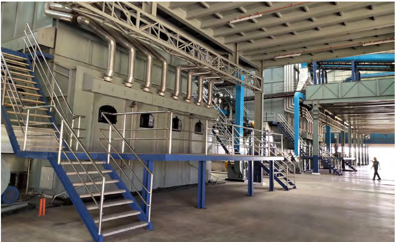
Biomass Reciprocating Boilers at the Optimill.
