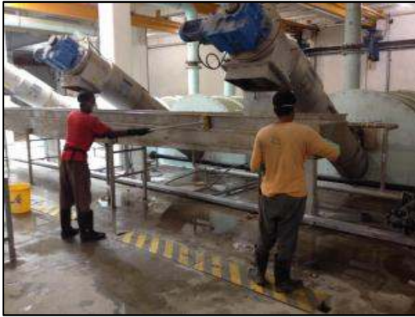
Kerja pembersihan 'Rotary Fine Screen'
