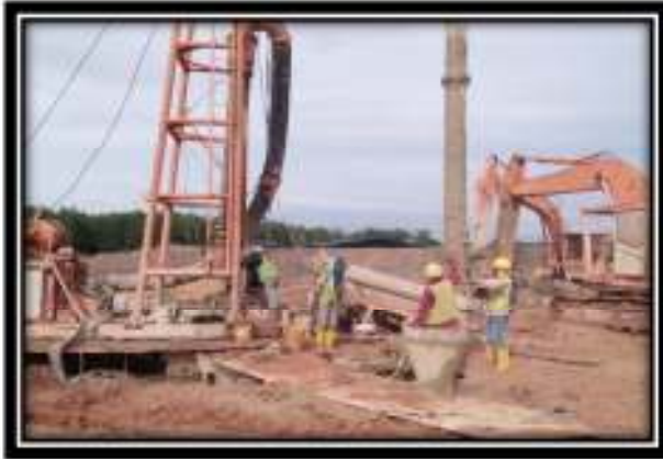
Kerja-kerja Penanaman Bored Pile
