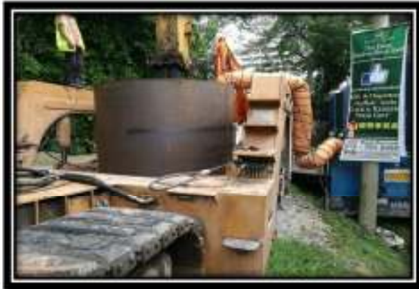
Casing Extraction
