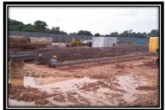
Besi tetulang Bored Pile
