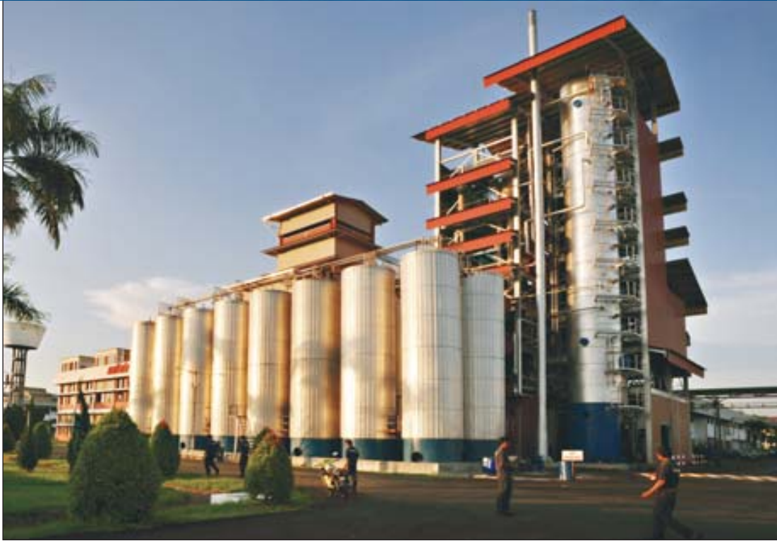
Multistock Deodoriser Plant at Unitata which was commissioned in 2009.
