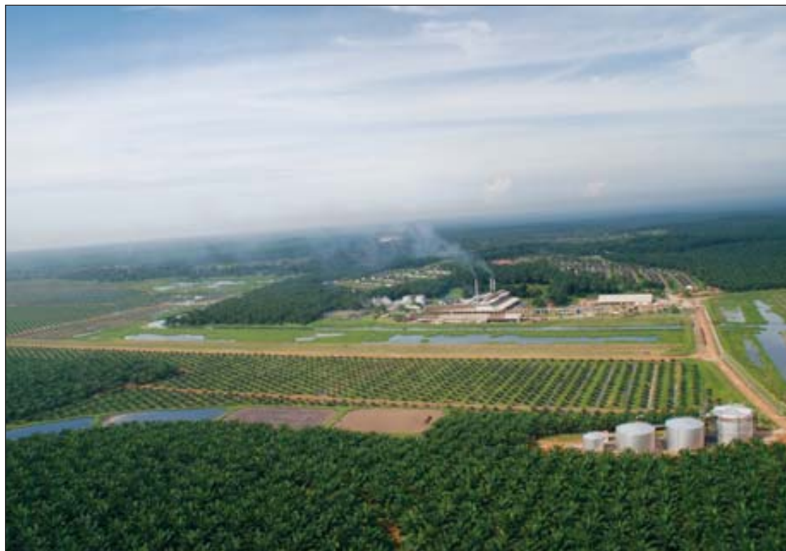
A third Biogas Plant has been built at Ulu Basir Mill to reduce carbon footprints.
