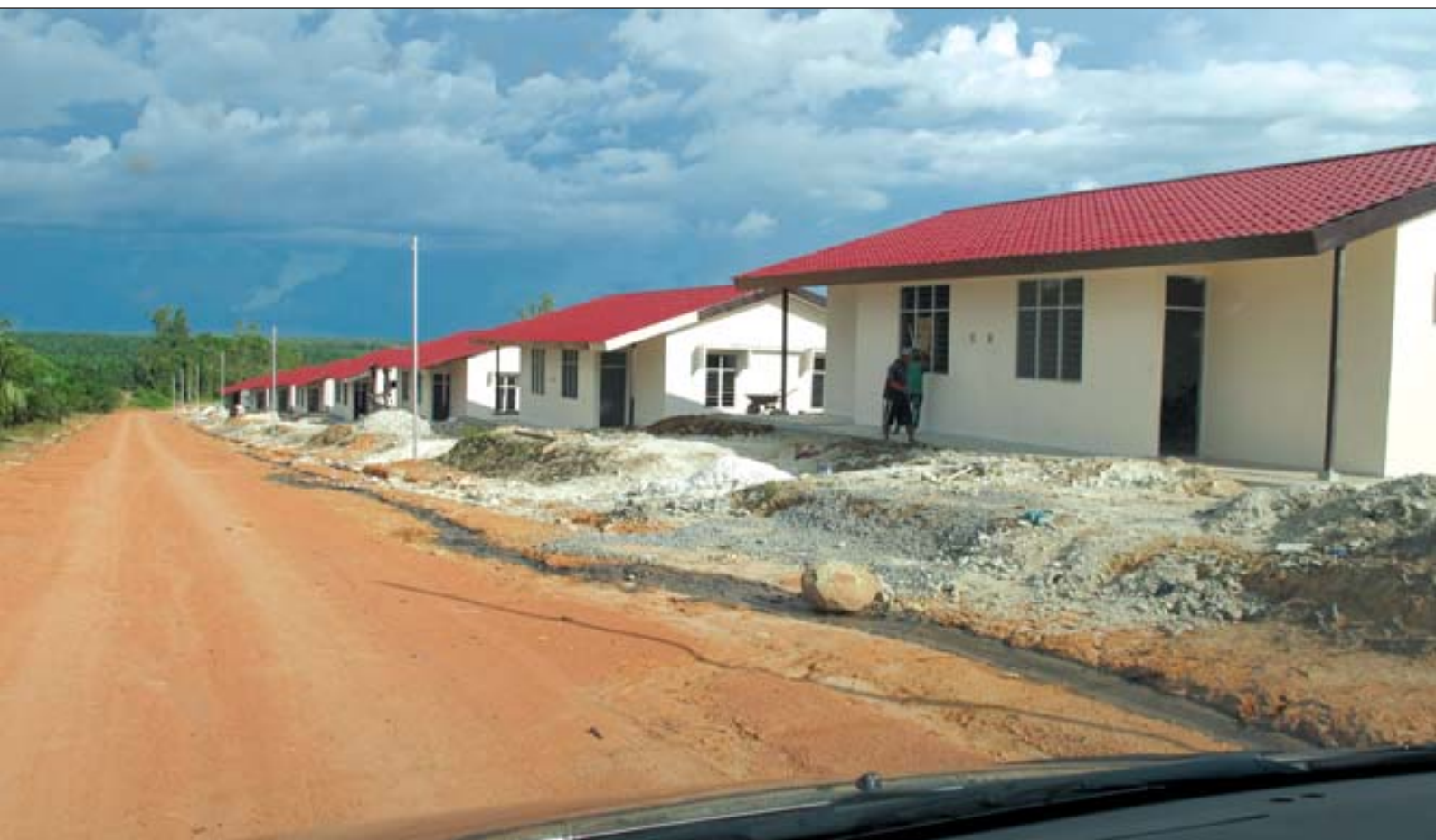
New housing complex at Lada Estate, Central Kalimantan nearing completion.
