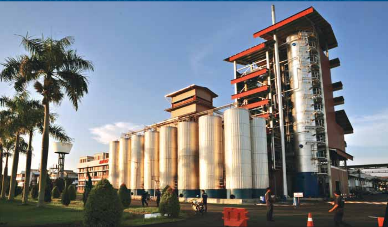
Multistock Deodoriser Plant at Unitata which was commissioned in 2009.
