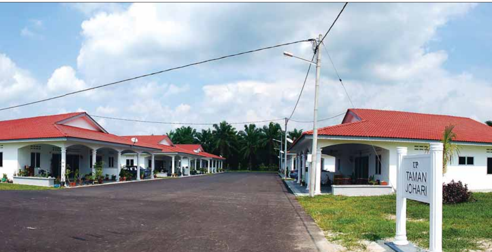
Recently completed workers' quarters with 3 bedrooms, a spacious living area and tarmac road access at Taman Johari, Jendarata Estate, Division 3
