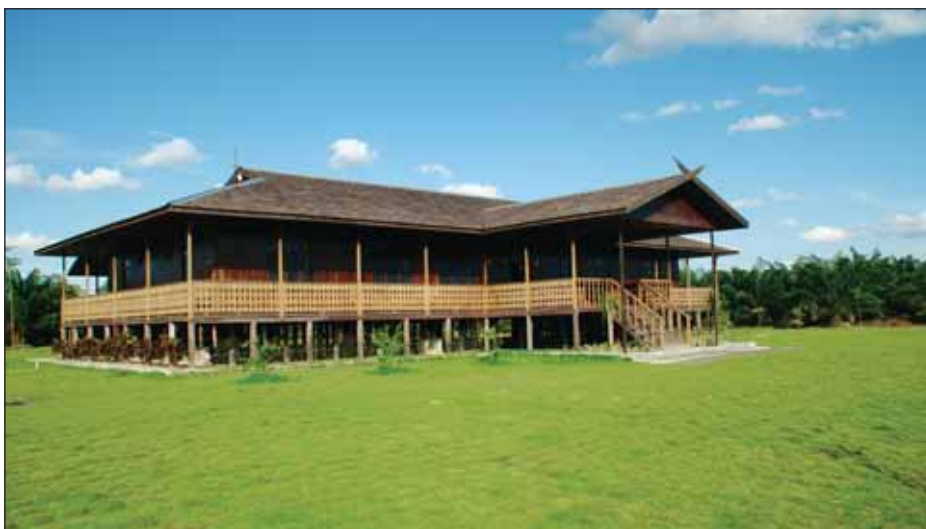
Our newly completed guest house of classical design to accommodate overseas visitors on business, built to blend with the natural surroundings at Lada Estate, Indonesia.
