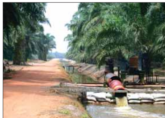
Water management activities within the estate.
