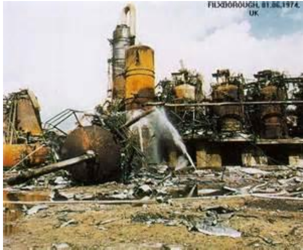
Flixborough (Nypro UK) Explosion 1st June 1974
