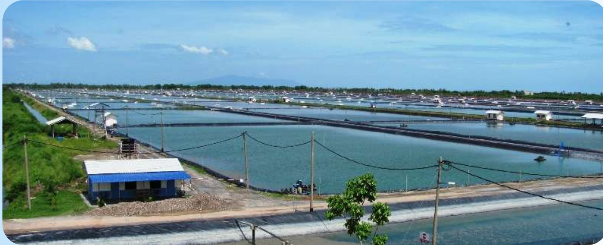
HDPE lined ponds with center drain, secured outlet gates & Main supply canal
