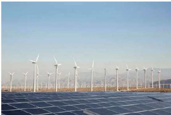
Wind Turbines and Solar panel Credit: www.nrdc.org
