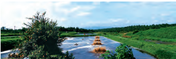
Palm oil mill effluent is treated using the pond systems before being discharged into the environment
