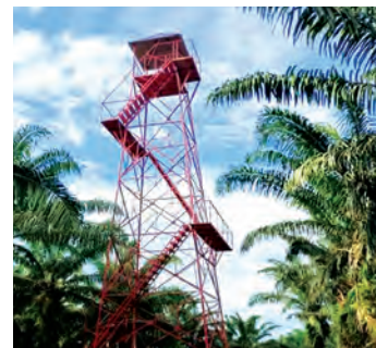
Fire tower was set up to inform ground patrol of any occurrence of fire
