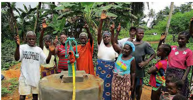
Provision of water pump to supply clean drinking water in Liberia
