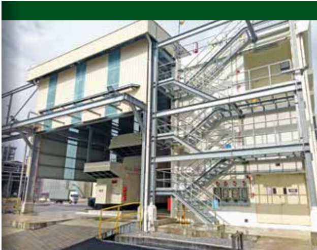
A new COGEN at Oleomas
