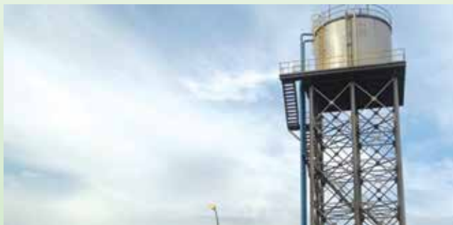
Water Treatment Plant at RSB Palm Oil Mill
