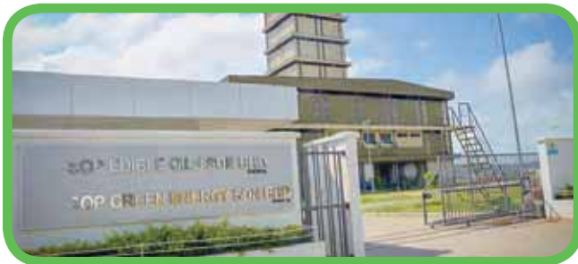
Gate entrance view with refinery building at the background
