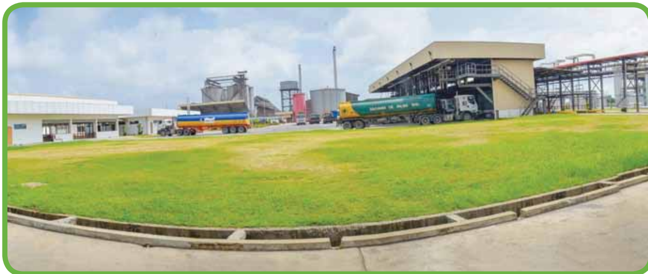
CPO Receiving and Loading Building
