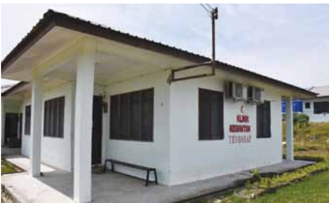
Health Centre are provided at certain estates to provide basic medication needs for the workers.
