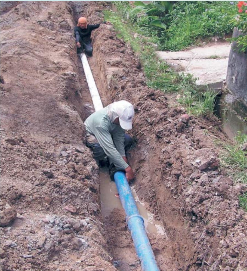
Pipe repairs and maintenance works for Sandakan NRW, Phase 1 Project.
