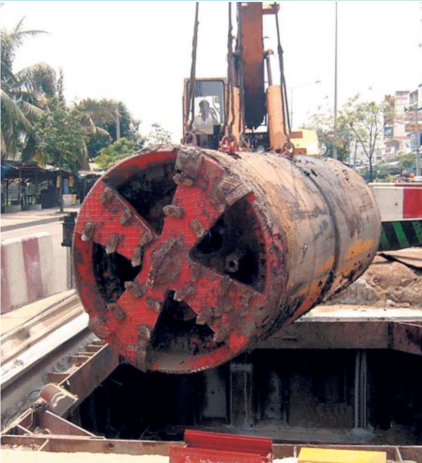
Pipe head jack works for PIT 711 project at Bangkok, Thailand.
