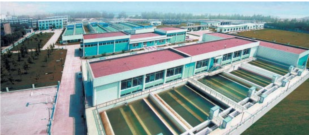
Aerial view of Linyi Water Treatment Plant.
