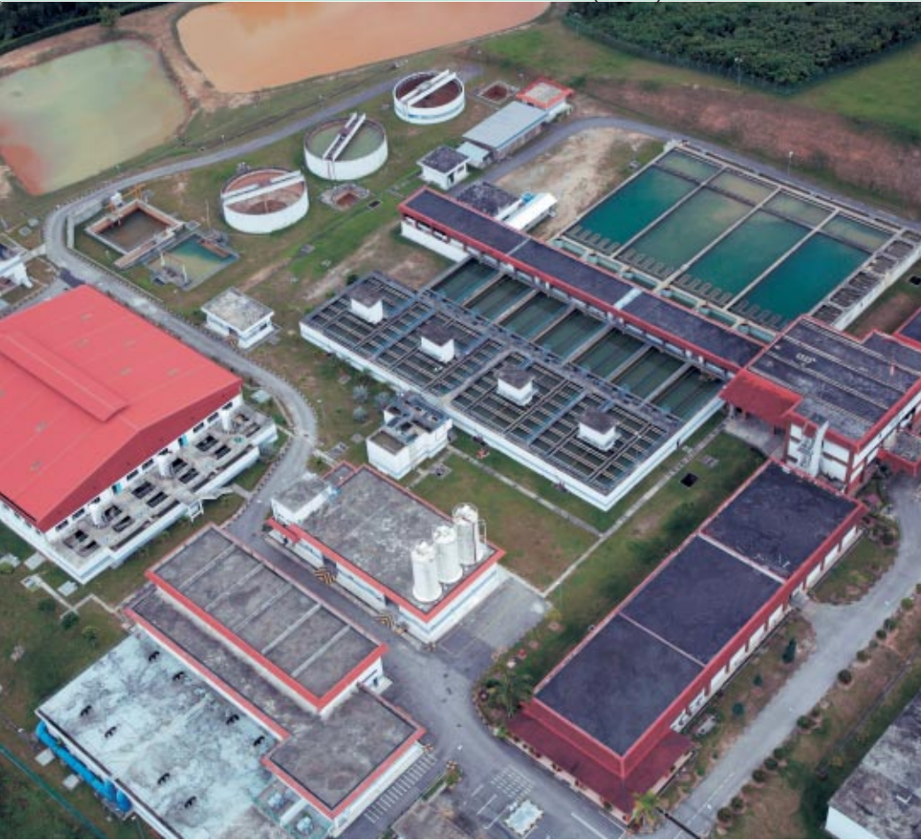
Aerial view of Sg. Terip Water Treatment Plant, Negeri Sembilan where Salcon is providing on-going operation and maintenance services.
