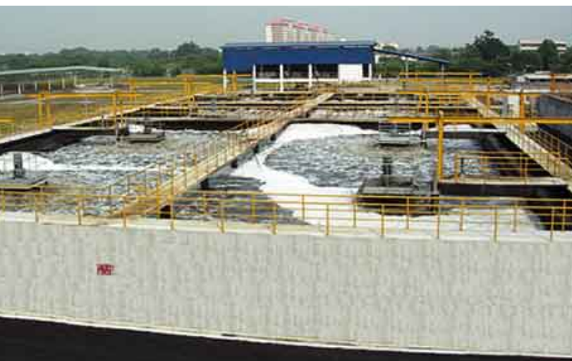
Regional Sewage Treatment Plant for mix development for Bandar Bukit Tinggi 2, Klang, Selangor (Module 2)
