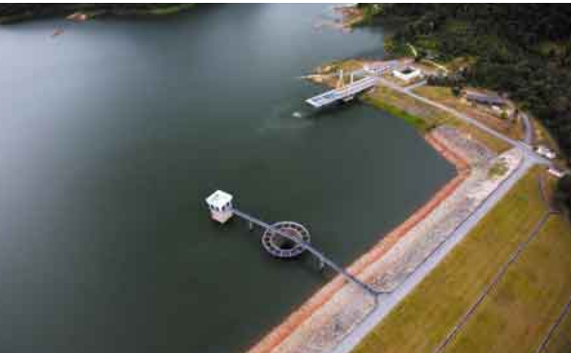
Aerial view of Sg. Terip Dam, Negeri Sembilan
