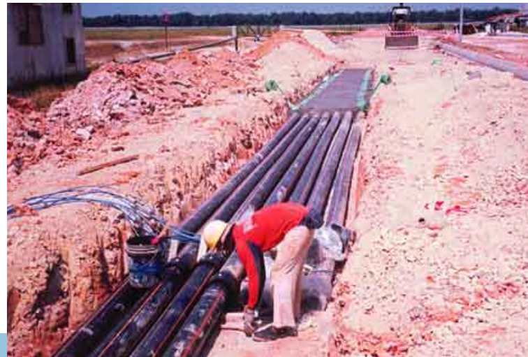
Vacuum/Gravity sewerage reticulation for Bandar Bukit Tinggi 3, Klang, Selangor
