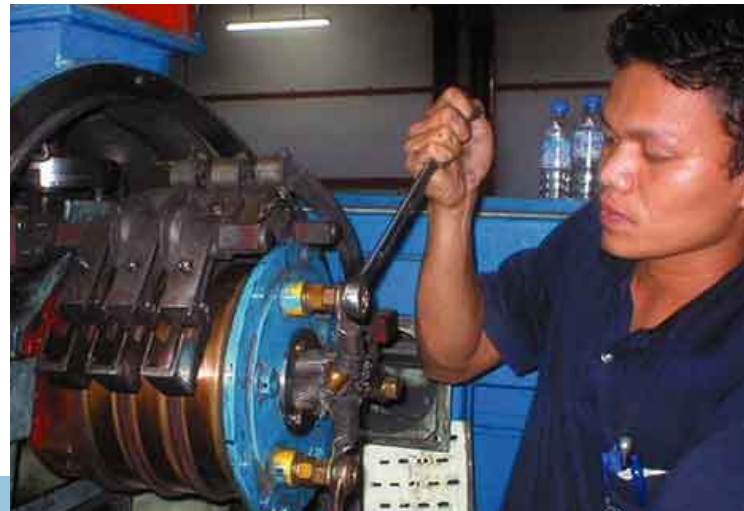
Regular preventive maintenance checks conducted at water treatment plants.
