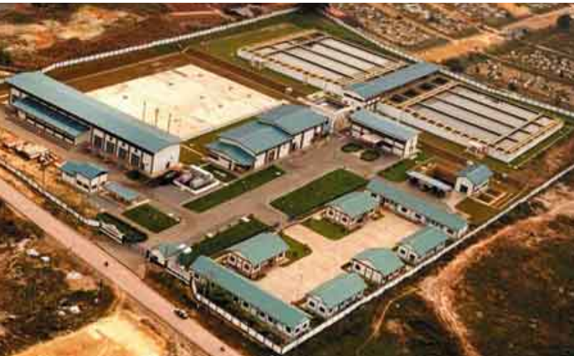
Binh An Water Treatment Plant in Ho Chi Minh city, Vietnam
