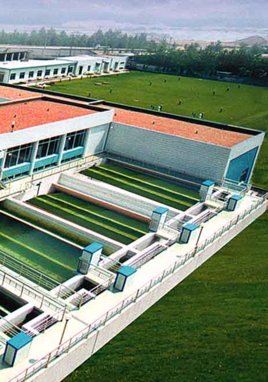
Overall view of Dong Bei Yuan Water Treatment Plant, Linyi City, Shandong Province, People's Republic of China
