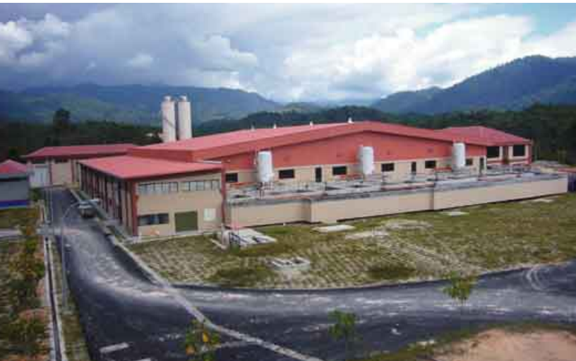
View of Sg. Kinta Water Treatment Plant
