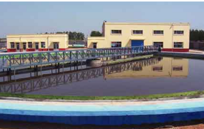
Changle Wastewater Treatment Plant, Shandong Province, People's Republic of China
