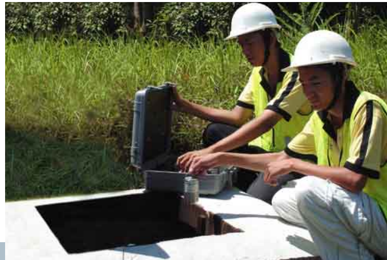
Installation of acoustic loggers in distribution system for leak detection
