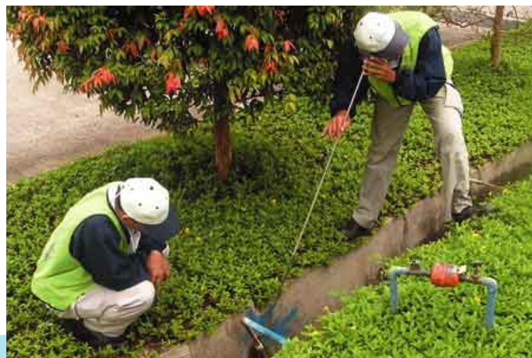
Detecting underground leaks
