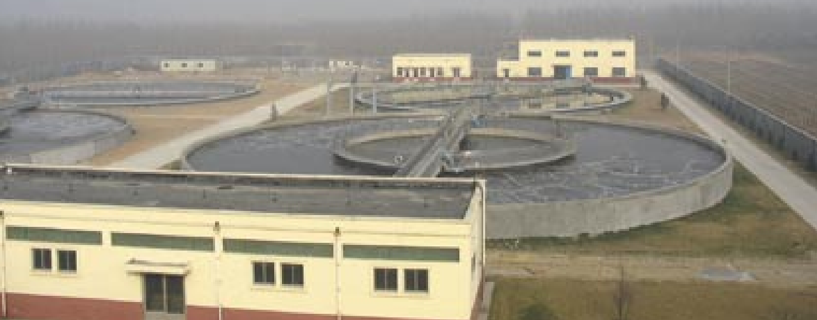
Wastewater Treatment Plant upgraded from existing 20 MLD to 40 MLD in Changle County, Shandong Province, People's Republic of China
