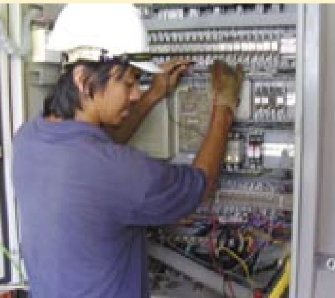
Stringent safety standards are practised to ensure a safe working environment
