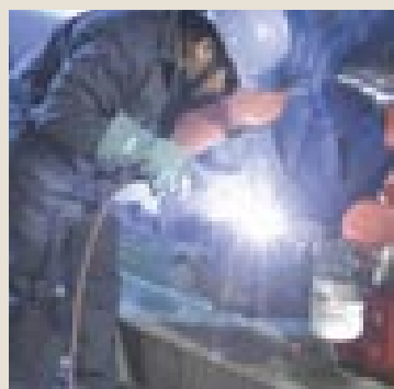
Repair and Maintenance works
