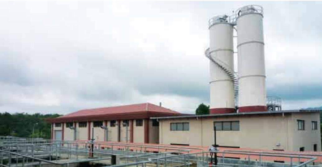
*View of clarifier tank and lime silo at Sg. Kinta Water Treatment Plant, Perak*
