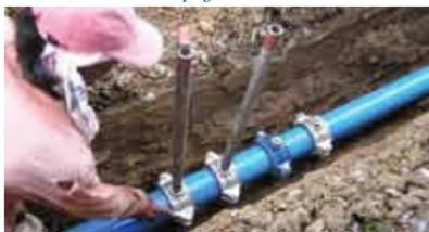
Fixing of saddle and ferrule for new tapping point
