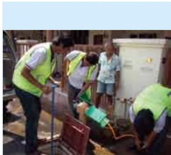
*Checking flow of meter in progress for Kelantan Non Revenue Water works*
