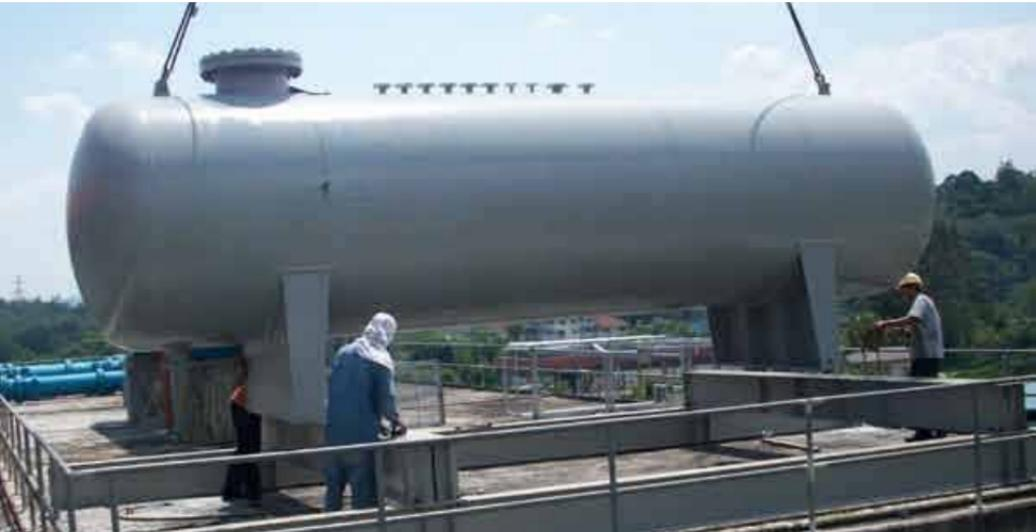
*Installation of surge vessel in progress to increase pumping and treatment capacity to Sg. Terip, Negeri Sembilan Water Treatment Plant*
