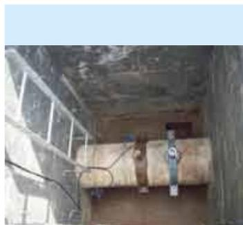
*Flow measurement using ultrasonic meter for Kelantan Non Revenue Water works*
