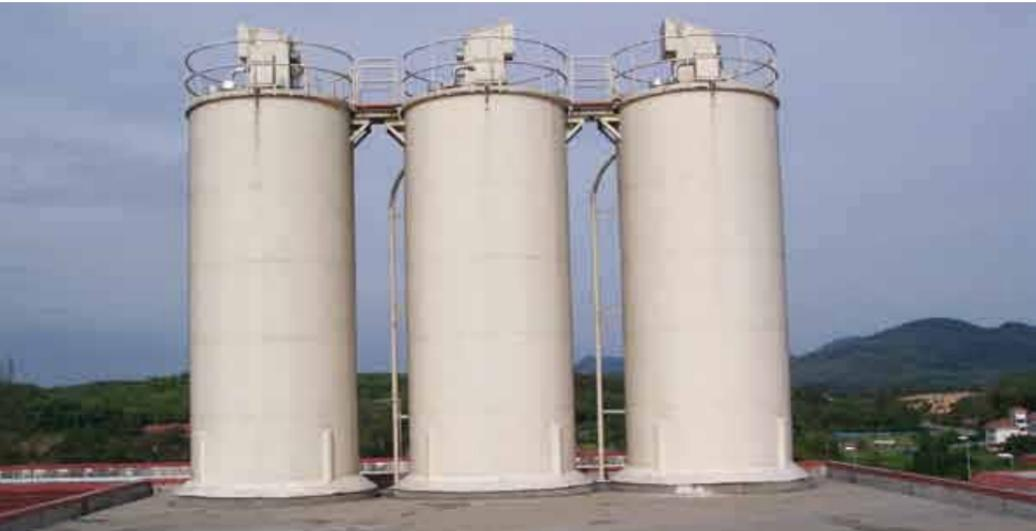
*Lime Silo with a capacity of 100m<sup>3</sup> each at Sg. Terip Water Treatment Plant, Negeri Sembilan*
