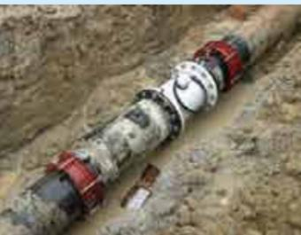
Installation of 300mm diameter battery powered flow meter production measurement for Seremban Non Revenue Water works, Negeri Sembilan
