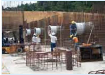
*Cast in pipe installation works at Raw Water Pumping Station for Teriang Water Supply Package 2, Negeri Sembilan*
