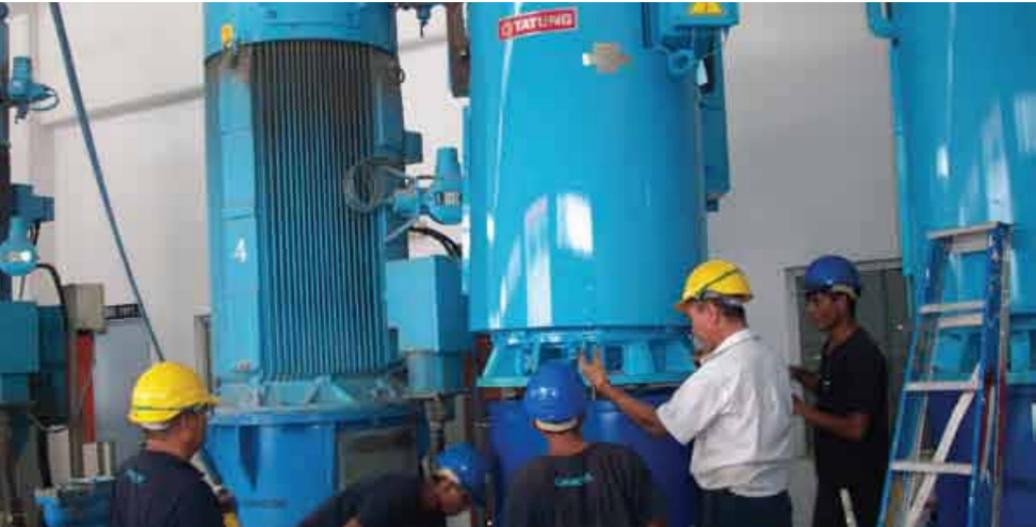
Installation of treated water pumps in progress to increase pumping and treatment capacity of Sg. Terip Water Treatment Plant, Negeri Sembilan
