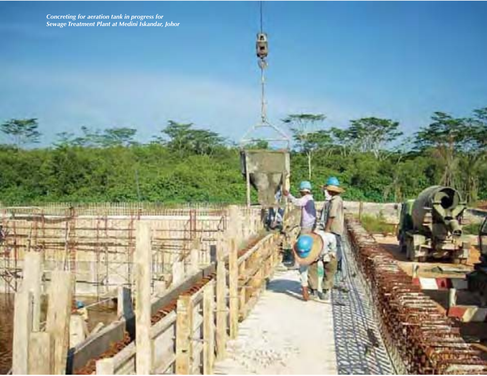
Fixing Rebar for biological treatment in progress for Sewage Treatment Plant at Medini Iskandar, Johor
