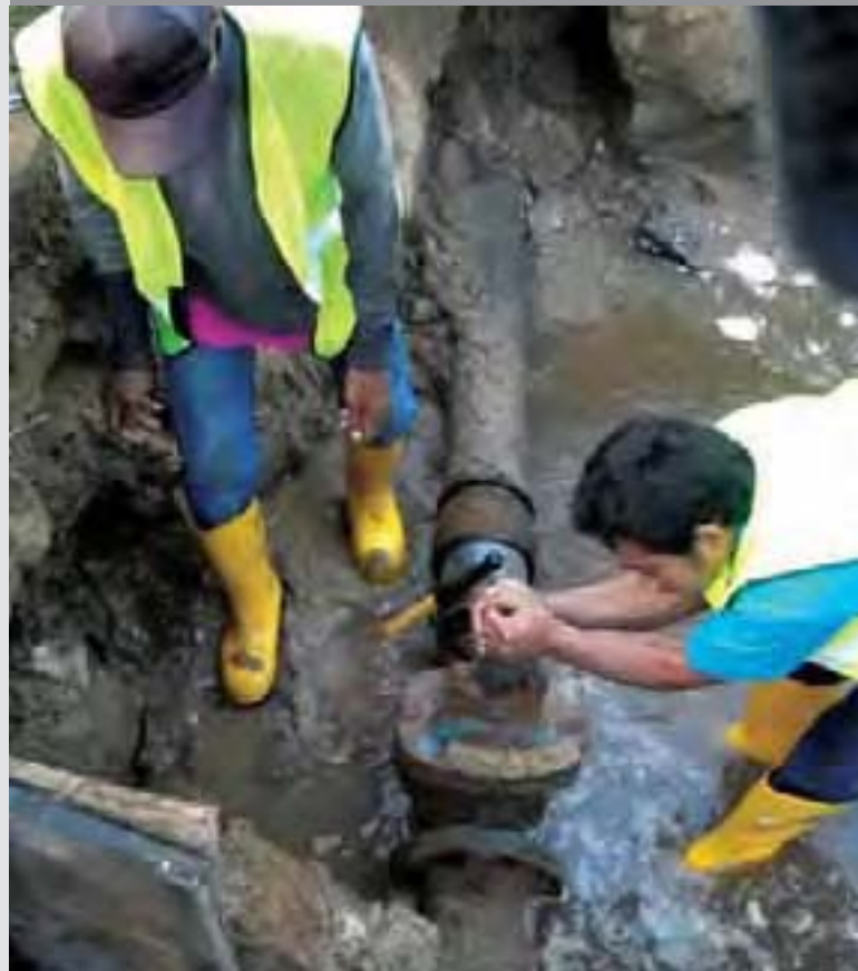
Leak repair works in progress for Kelantan NRW works
