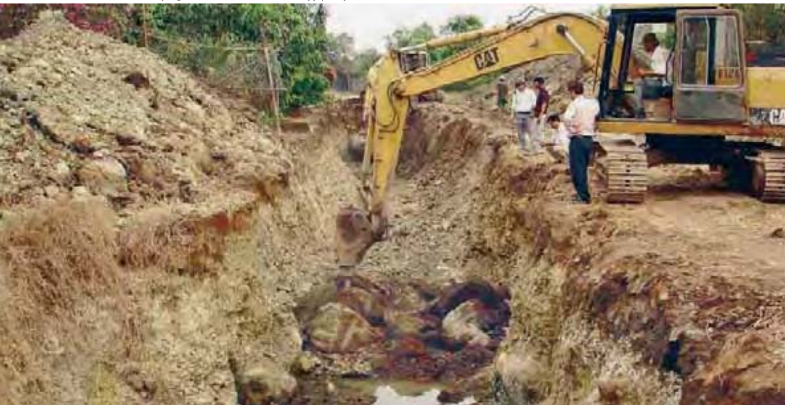
Excavation works in progress for Nhon Trach Water Supply Project, Vietnam
