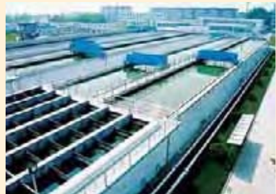
Linyi Water Treatment Plant, Linyi City, Shandong Province, China
