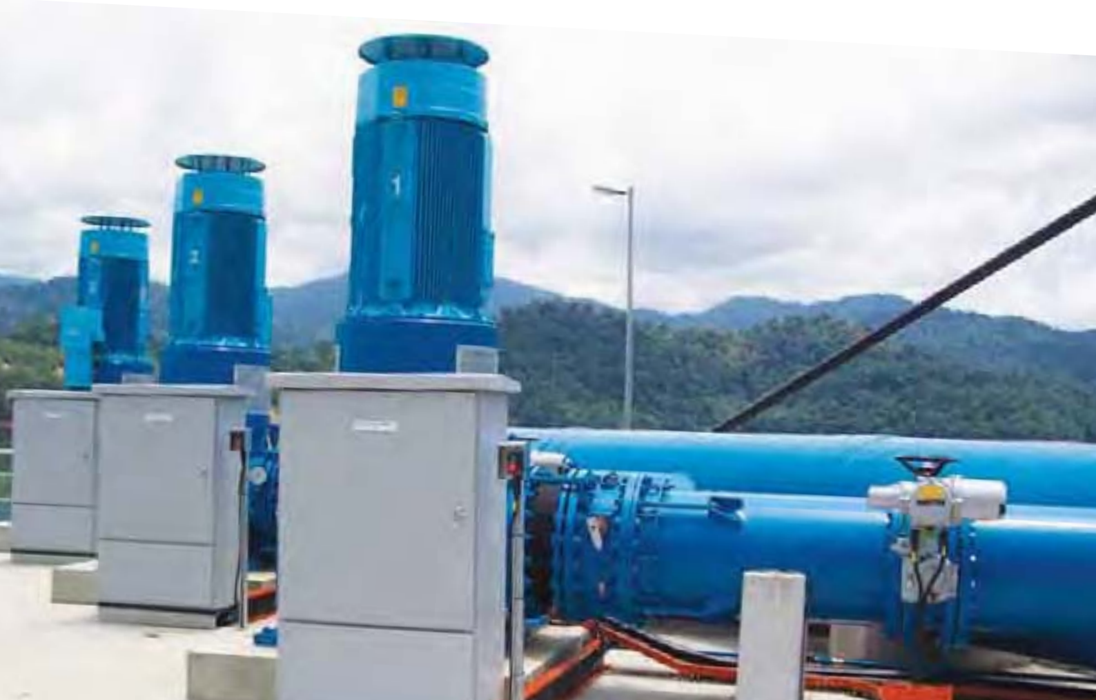
Dam draw off vertical turbine pump with a maximum capacity of 25 million gallons per day at Sg. Terip water treatment plant, Negeri Sembilan
