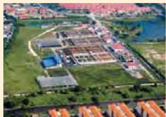
Aerial view of Bukit Tinggi Sewage Treatment Plant, Klang, Selangor
