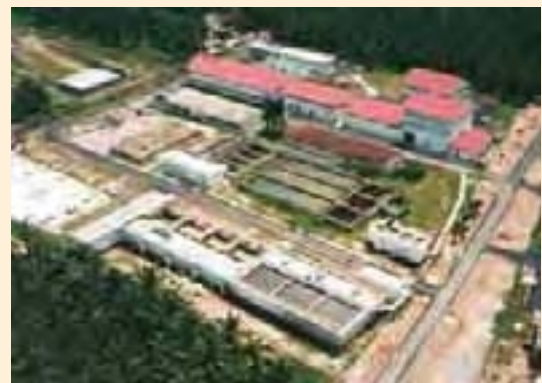
Aerial view of Kuala Jelai Water Treatment Plant, Negeri Sembilan
