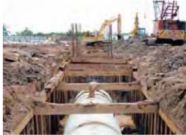
Raw water pipe laying works at Dong Tam, Vietnam
