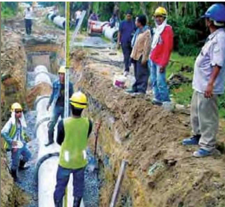
View of pipe laying work with proper bedding for Kota Kinabalu sewerage works Phase 1, Sabah
