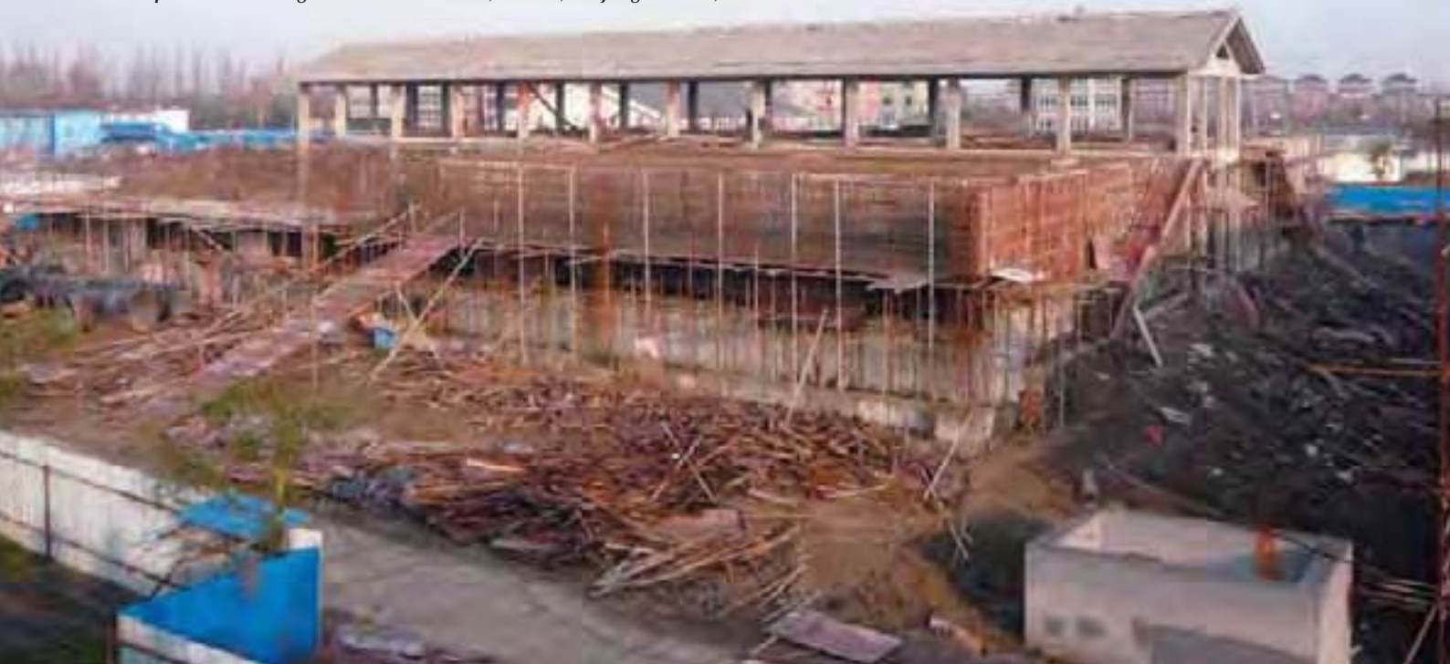
Expansion of Haining Water Treatment Plant, Phase 2, Zhejiang Province, China
