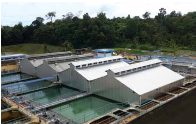
View of 120MLD Sg. Lebam Water Treatment Plant and distribution system in Johor was completed within schedule.
