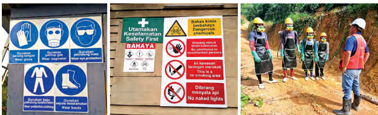
Appropriate safety signages are installed and PPE is provided to workers
