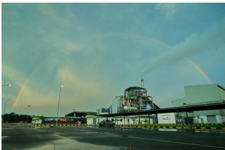
MJE announced the grand opening of its RM 160 million, ISO-certified, first of its kind, large-scale, advanced clean energy technology biomass power generation facility
