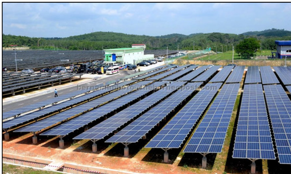
The Amcorp Gemas 10.25MW Solar Power Plant in Gemas, Negeri Sembilan
