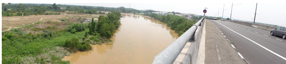
Sedimentation in Sg. Langat causes the water to be shallow at the Banting Bridge in Mukim Tanjung Dua Belas, Kuala Langat
