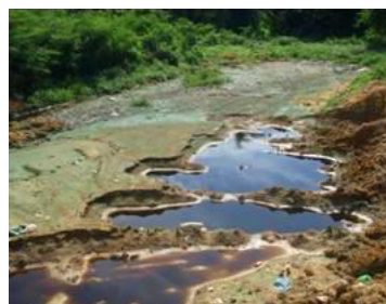
A bund failure at the Pajam landfill causes leachate to seep into the river Source: LUAS 2012
