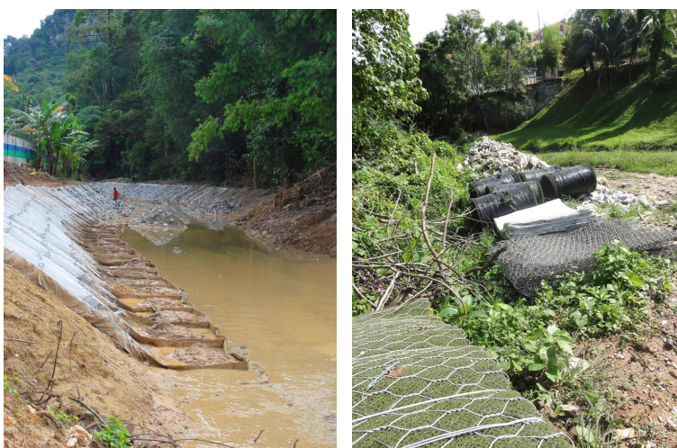
Cells for vegetating the banks of Sg. Klang; terramesh being installed along the banks
