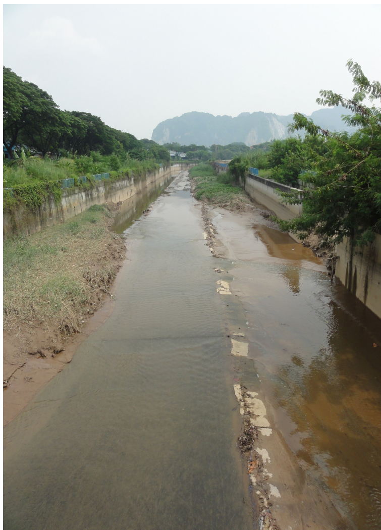
The Gombak Diversion helps prevent river breaching of Sg. Gombak by diverting excess stormwater to Sg. Batu
