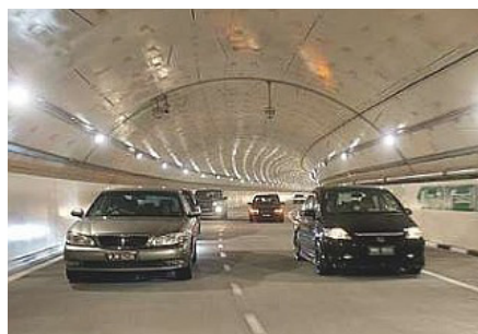
A two-level motorway and a third level for stormwater conveyance Source: JPS
